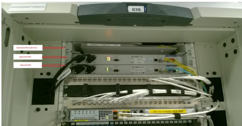
2x 1U Openreach NTES in a customer cabinet
